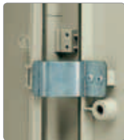
Anti-lever security system.
