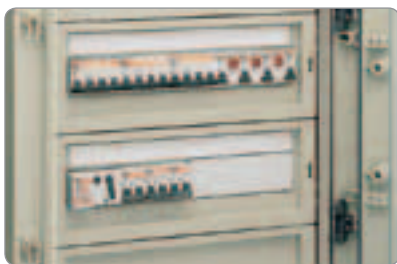
Detail from the circuit-marking system.
